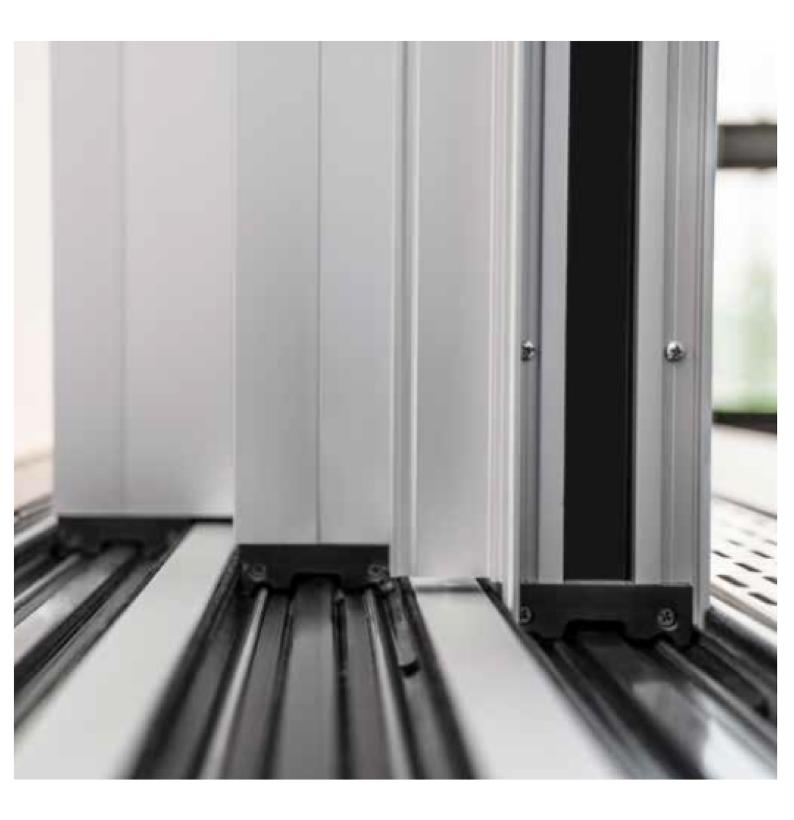
3 | Any foreign bodies that obstruct water drainage in the floor track must be removed immediately in order to prevent damage. The same applies during the winter months: Ice and snow can also prevent water drainage, and must be removed from inside and in front of the floor track.
